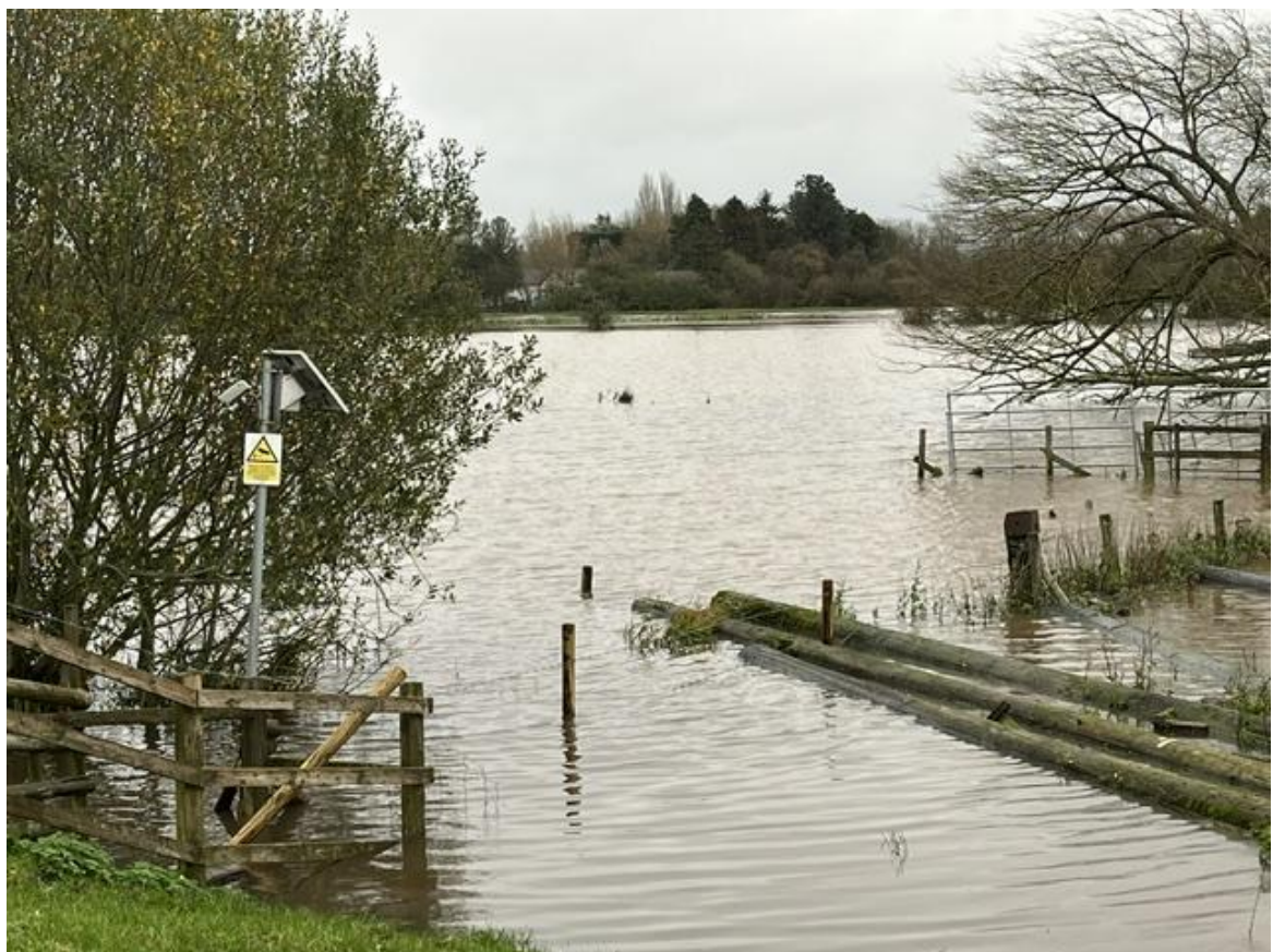
Figure 2.2: Site E from Egginton Flood Defence Bank
