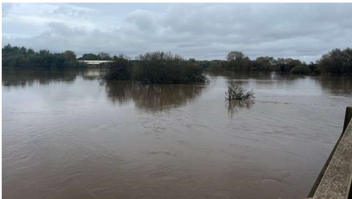
Figure 2.3: Site E from the A38 looking west - flood of 2022 showing the STW abstraction plant
