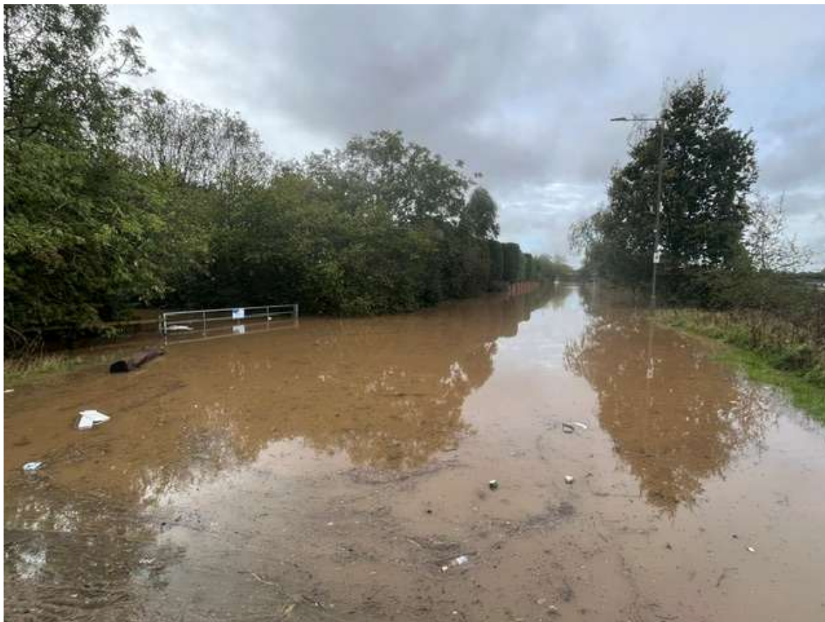
Figure 2.1: Church Road Egginton under flood - proposed access to site showing extent of flood at Egginton Church Road Sewage Pumping Station (SPS)
